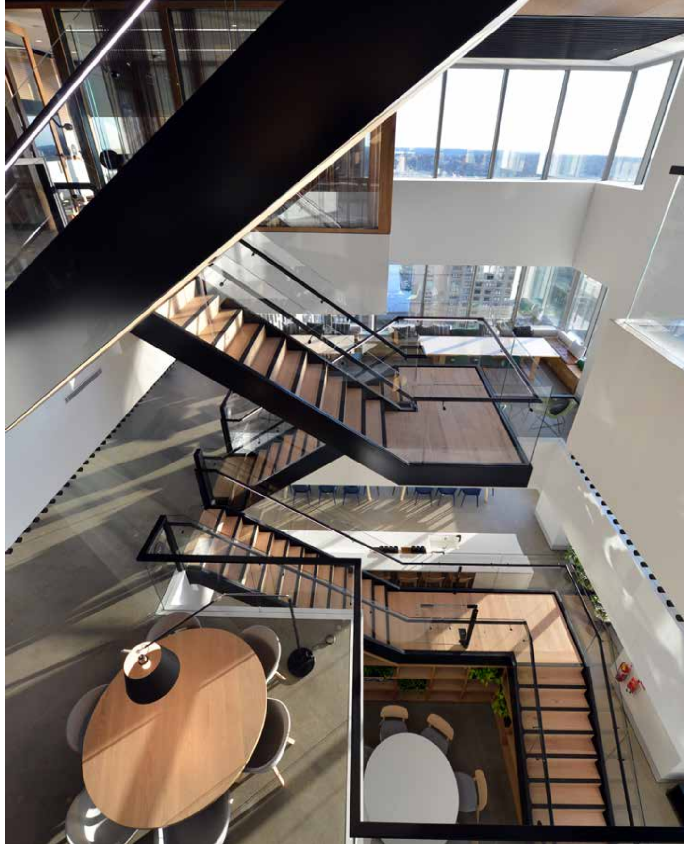
A new void for the stairs is cut into each floor
